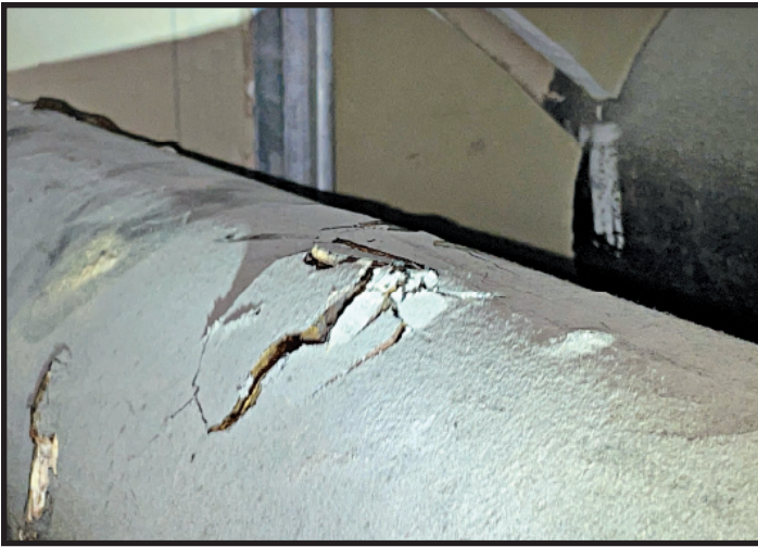
Shown here are examples of cast iron kitchen waste piping that demonstrate failures resulting in the process described in this article.
